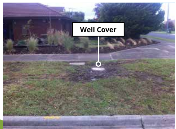
Completed Drill Hole, 14 Nov
