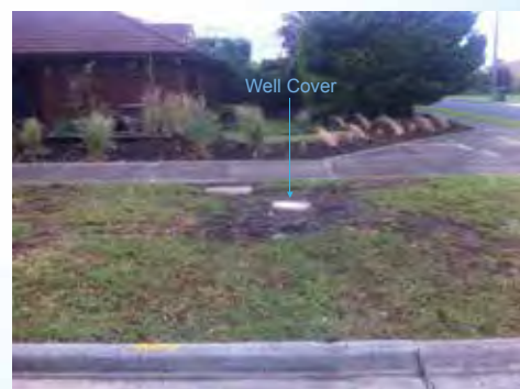
Completed Drill Hole, 14 Nov
