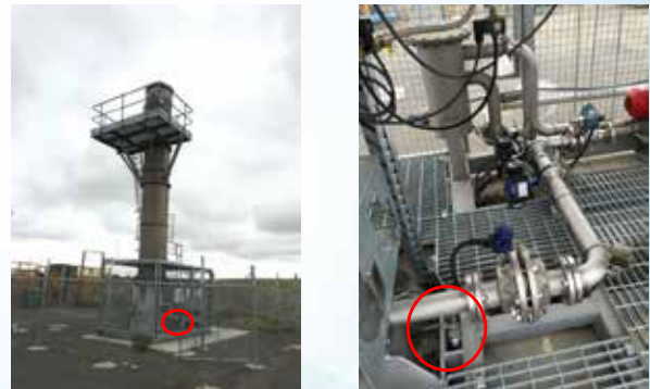
Flare Equipment (new sample locations circled in red)
