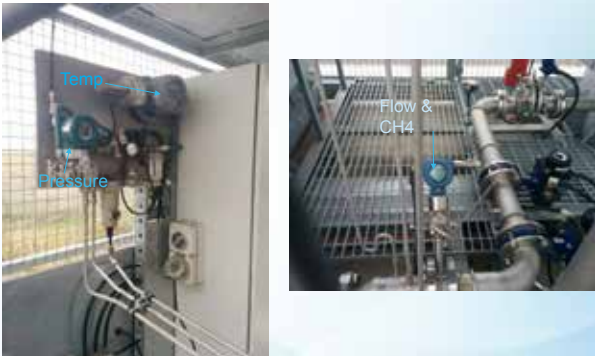
Flare Sampling Equipment - Calibrated In-Situ Equipment Methane (CH 4 ), Temp, Pressure, Flow
