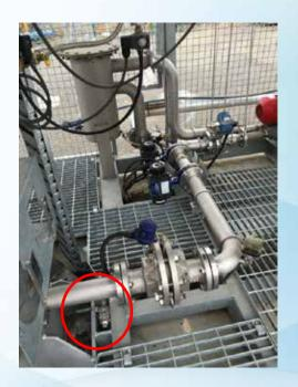
Ektimo used the sampling points shown to collect samples directly into a canister which reduced contamination or air exposure.
